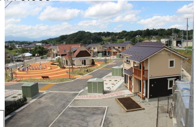
litate village disaster recovery public housing - lino-machi housing complex (Fukushima city)
