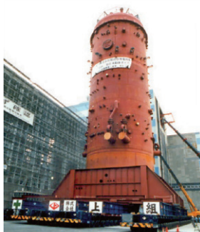
Transportation of Pressurized Fluidized Bed Boiler (3,820 tons) for a Thermal Power Plant
