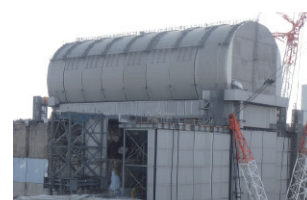
Fukushima Daiichi Unit 3, engineering and construction of cover structure for fuel removal (as of February 2018)
