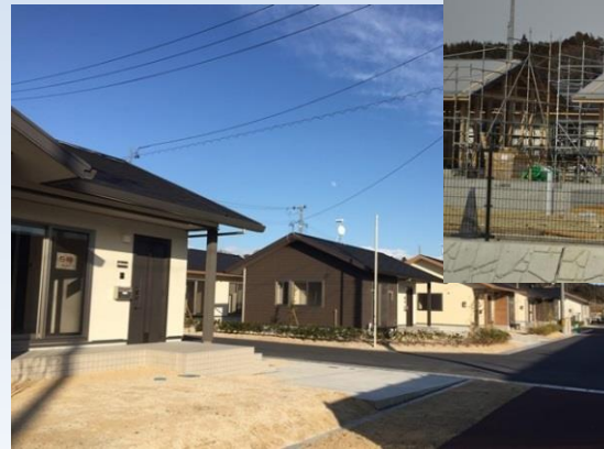
Public restoration housing (move-in began in Nov. 2016)
