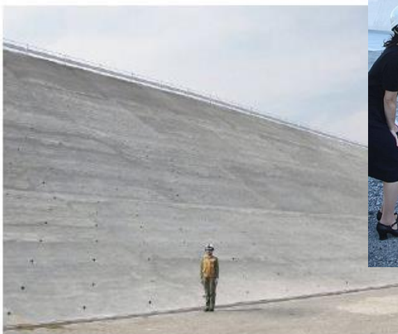
Cement-mixed soil embankment
