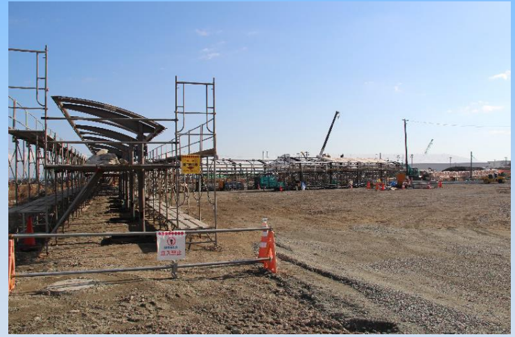
Station square to be completed in 2017 spring
