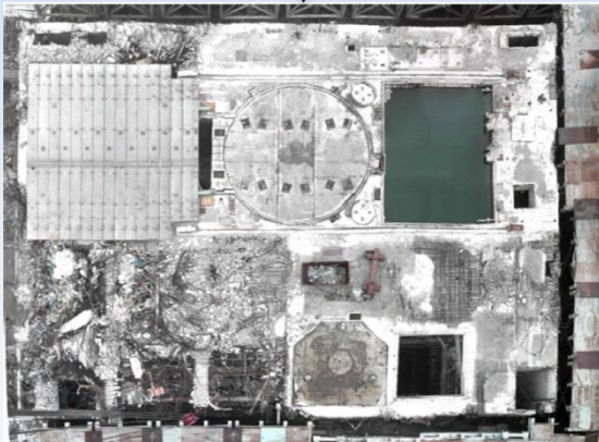
Unit 3 Operating floor, Mar. 2016
