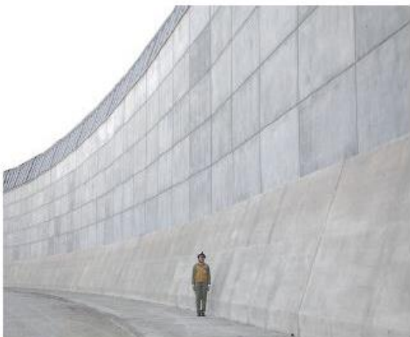
Tsunami protection wall (22m)
